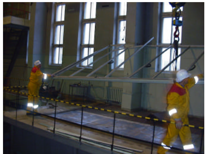
Fig. 3.6 Dismantling of unused computer building in reactor hall
