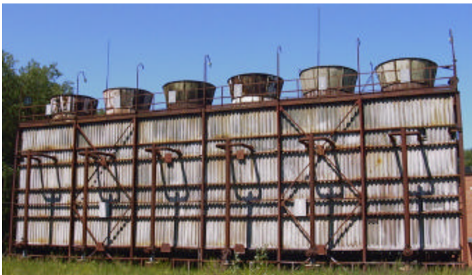
Fig.3.2. Reactor's cooling tower in July 1999.
